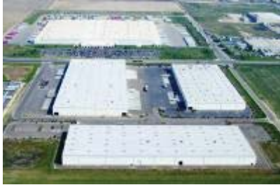
MidState 99 Distribution Center (Photo from The Allen Group)
